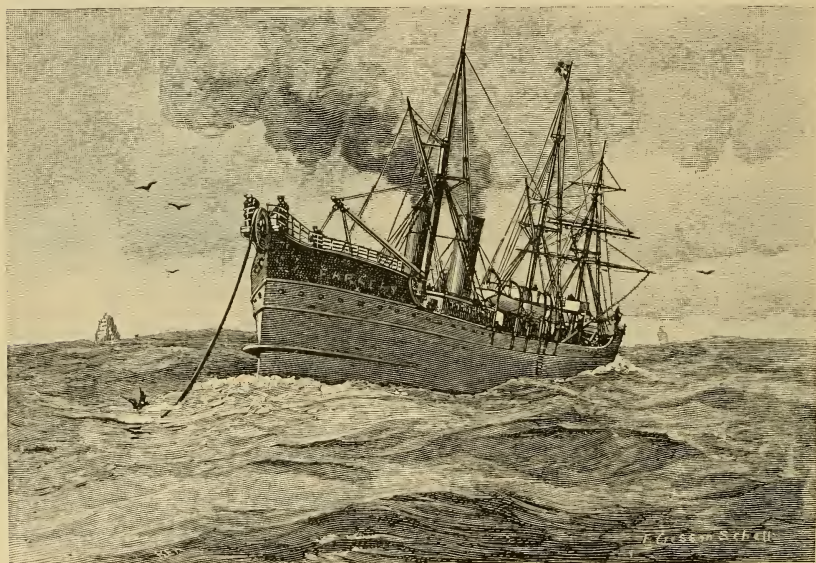
Laying an Atlantic Cable.
